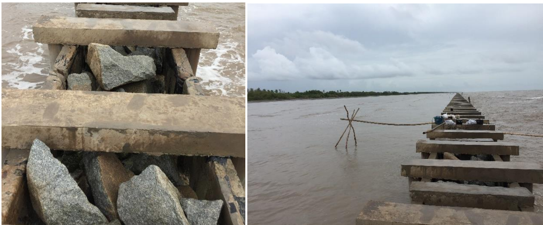
Figure 42: Example of existing concrete pile breakwaters in Ca Mau (July 2017).
