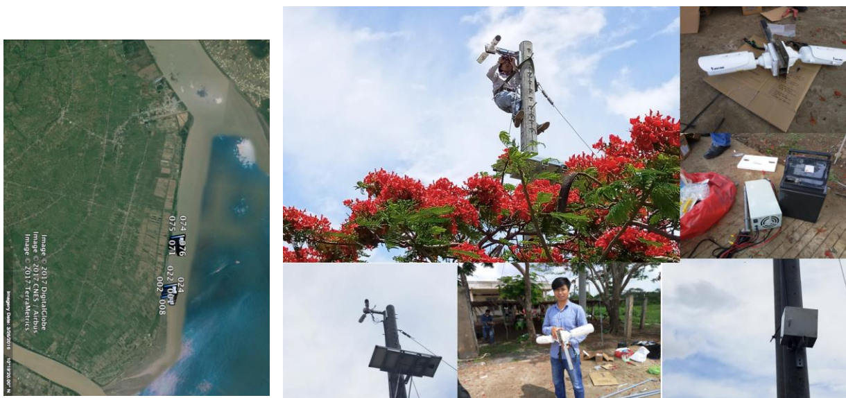
Figure 8: Installation of video cameras at Go-Cong on two poles each hosting 2 cameras
