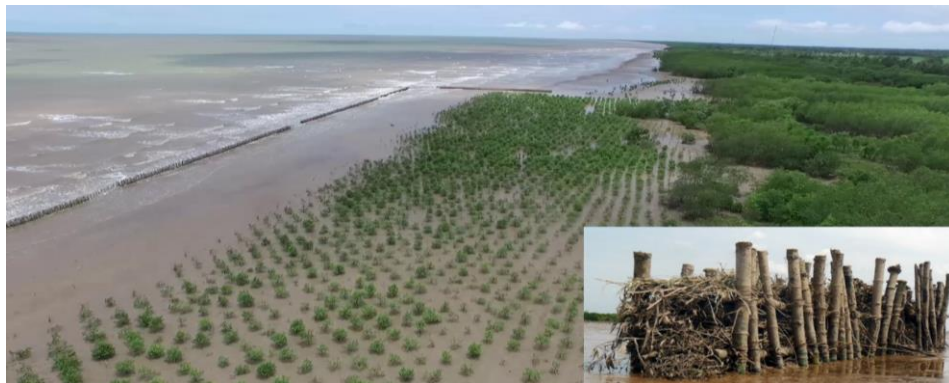
Example of soft structures: mangroves planting protected by wood/bamboo fences in Ca Mau
