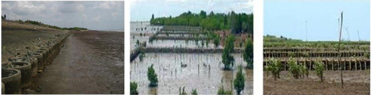
Figure 2-2 Foreshore erosion at Go Cong Revetment (left) and wave and current attenuation by T fences at Soc Trang and Bac Lieu provinces by GIZ projects [4]
