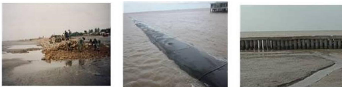
Figure 2-1 Breakwater by riprap (at Can Gio), geotube ( at Bac Lieu), and concrete piles (at Ca Mau)[4]
