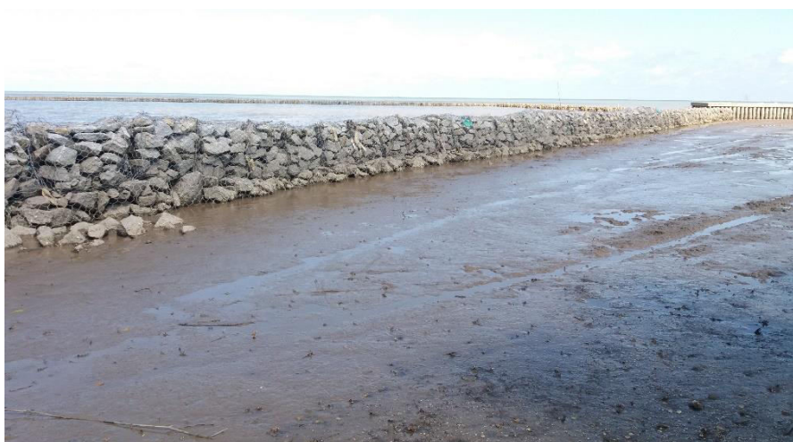
Figure 8. The foundation of mudflat inside concrete piles at Sao Luoi canal
