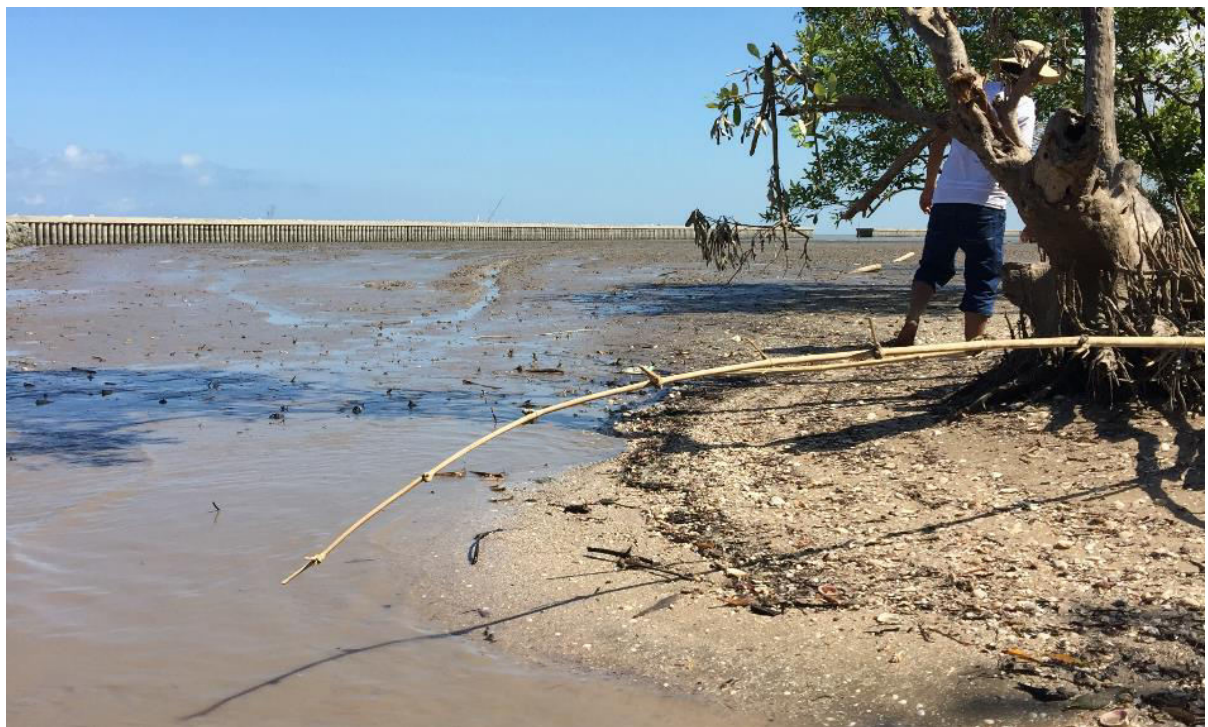
Figure 5. The topography of mudflat inside concrete piles at Sao Luoi canal
