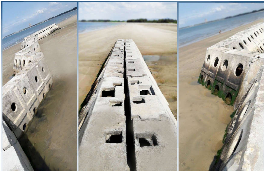
Figure 1 Pilot project of porous detached breakwater at Long Hai beach (Ba Ria Vung Tau province)
