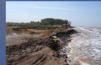
Revetment built along old dyke line and new dyke set up - 150 m far from old dyke line - 2009
